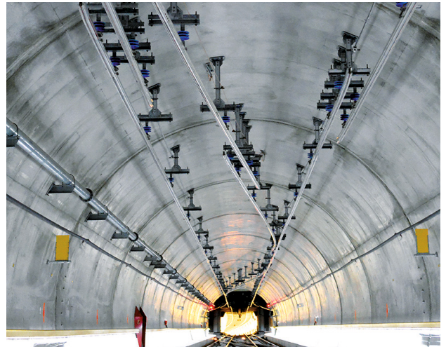
TracFeed® OSS Overhead conductor rail
