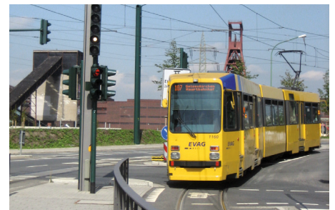
Catenary systems – with architecturally adapted design
