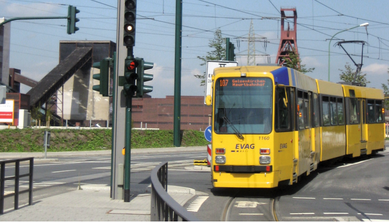
Contact line systems – designed as overhead line
