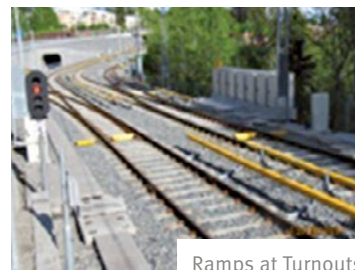
Ramps at Turnouts
